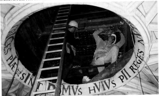
Fig. 10 Insulation being installed under the bell tower floor at Winchester Cathedral Rockwool Ltd
